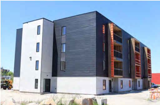
27-unit apartment building on Water Street
