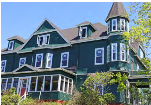
8 James Street will be 12 mixed-income units
