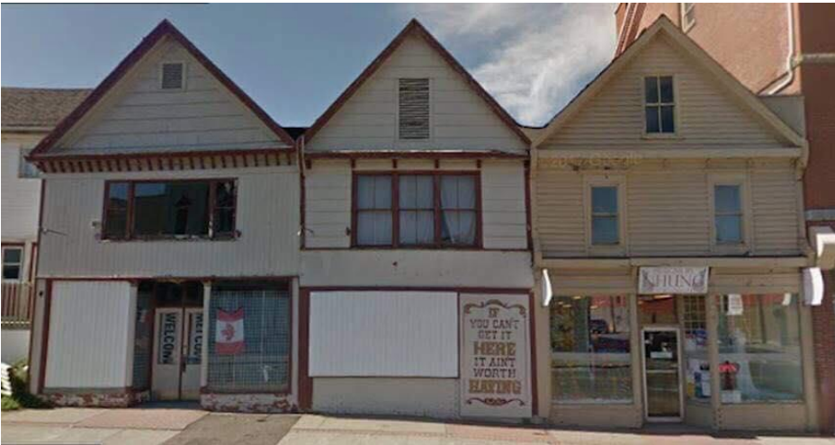
Before Photo 258 to 262 Main Street
