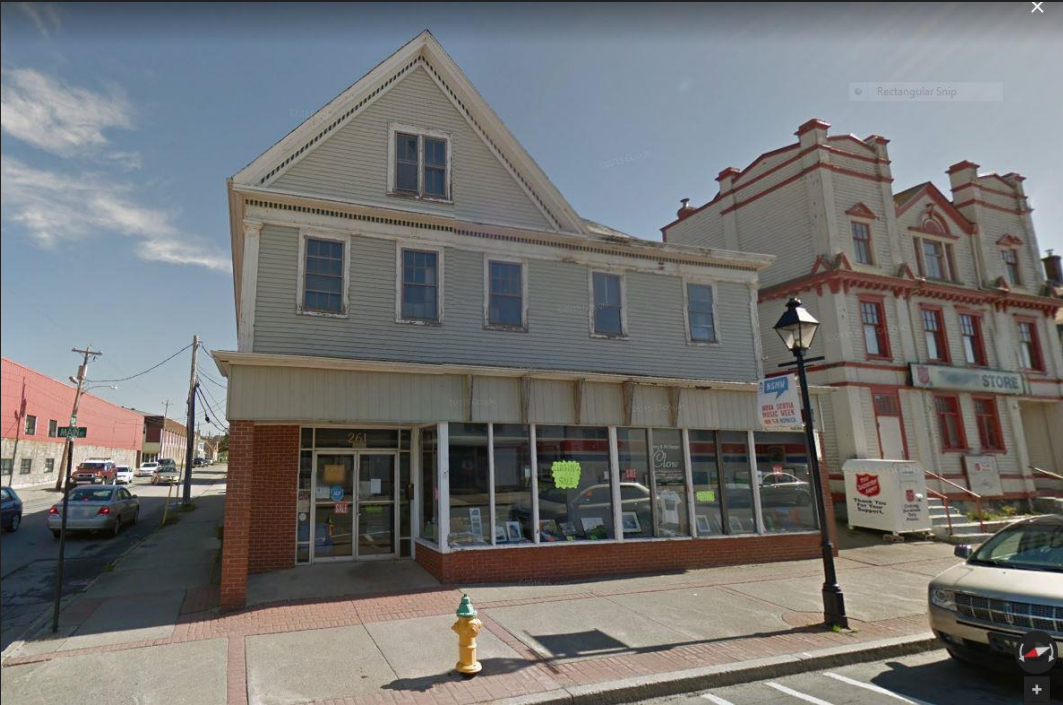
Current Façade 261 Main/ 9 Cliff St.
